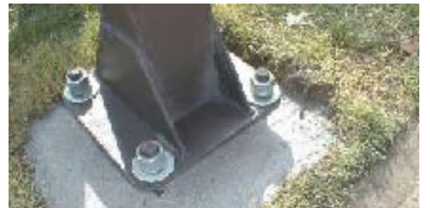
Figure 12 Adjust The Insert Nuts
