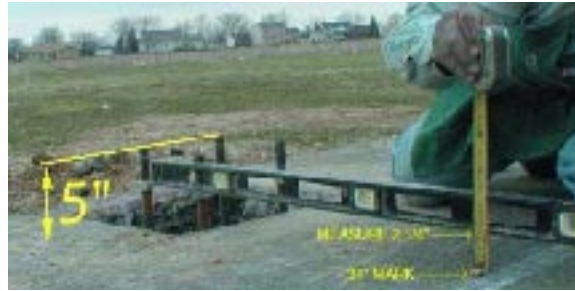
Figure 5 Measure Insert Depth
